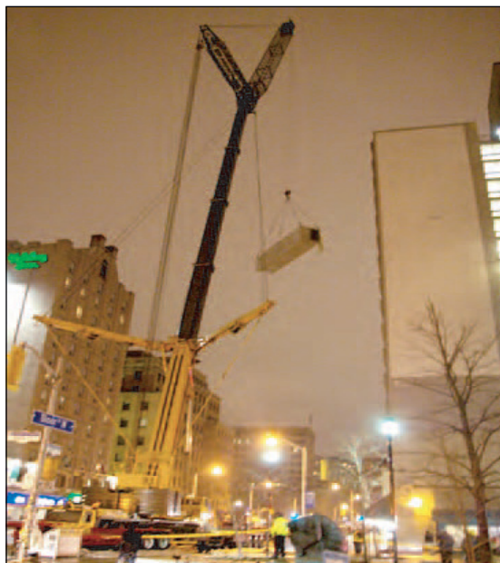
CHP Container Lift
