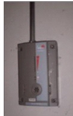
Top left: Parking garage lighting; top right: DHW boilers; above: CO monitor
